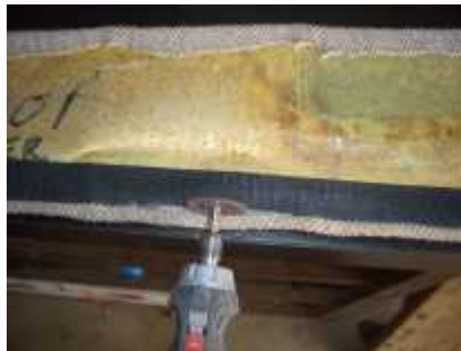
10. Slotting Interior panel.
