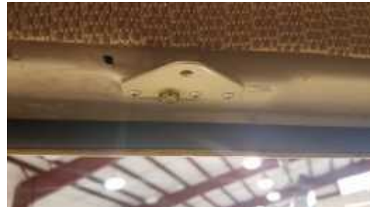
Picture 15. Door Bracket attached
