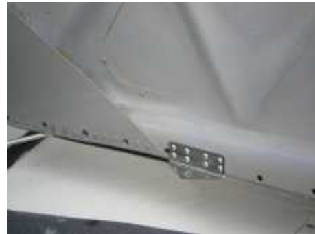
Picture 6. Door Bracket Installed
